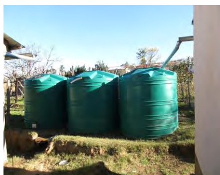
Fig 4.9: Installed plastic rainwater harvesting tanks at one of the homesteads in Nyanga, Cata Village
