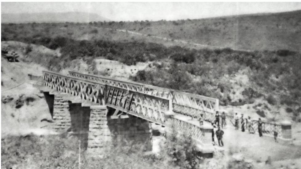
Fig 30: The re-constructed Cookhuis Bridge, showing one iron span and two timber spans
