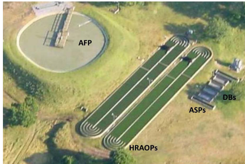
Figure 5 An aerial photograph of the IAPS pilot operating at the Belmont Valley WWTP treating 75 kℓ.d -1 municipal sewage. The pilot is composed of an AFP: Advanced Facultative Pond, which is a combination of an I-PD and a primary facultative pond, 2 HRAOPs: High Rate Algae Oxidation Ponds, 2 ASPs: Advanced Settling Ponds and 2 DBs: Drying Beds. Note the absence of an MP required for post treatment.
