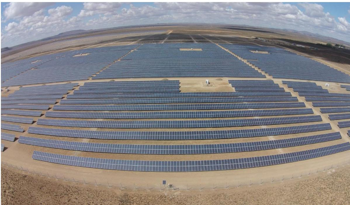
Figure 1.3: Solar Capital's De Aar PV plant, in South Africa, having thousands of crystalline PV modules [13].
