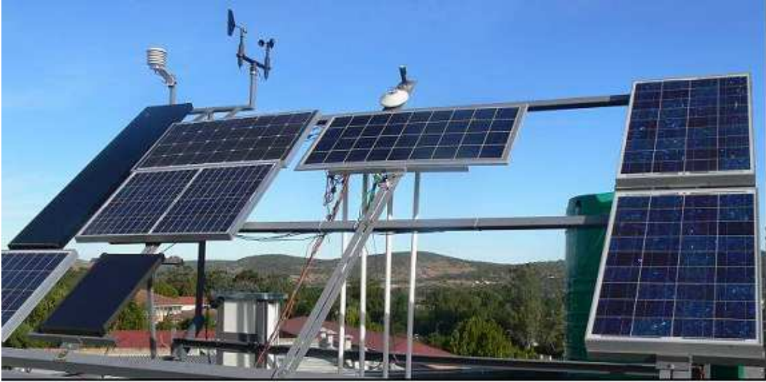
Figure 5.1: PV module layout installed at the Institute of Technology, South Africa at tilt angle of 32^{\circ}47' facing north.
