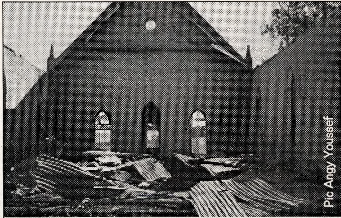
Interior of the building where wooden floors assured the flames spread throughout
