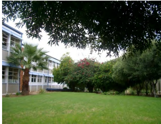
Picture 3: Garden facing the administration block
