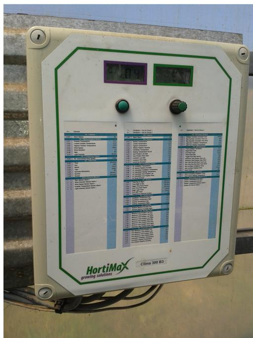
FIGURE 3.7: Hortimax Reading and Programming Interface (Hortimax, 2015)
