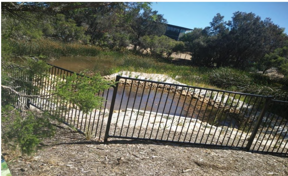
Figure 1-3. A picture of a FWS CW designed to treated storm water in Western Australia, Perth. The picture was taken during a field trip at the 2015 SWM conference in Perth, Australia.
