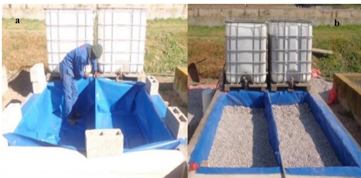
Figure 2-2. Construction aspects of V-H SSF hybrid CW. Lining the HSSF CW with PVC (a) hybrid CW filled with gravel (b)
