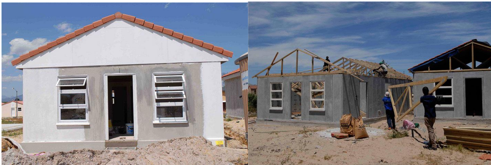
Figure 4.11: (a) Plastered walls and (b) Roof installation on complete modular shell (Concretex, 2019)
