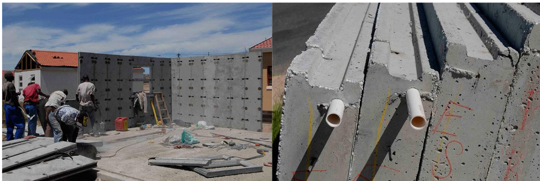
Figure 4.10: (a) Concretex Building System and (b) Conduiting cast into panels (Concretex, 2019)
