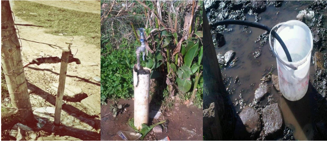
FIGURE 6.1 LEAKAGES AND BROKEN TAPS THAT ARE COMMON WITHIN NOMATHAMSANQA AND AQUAPARK
