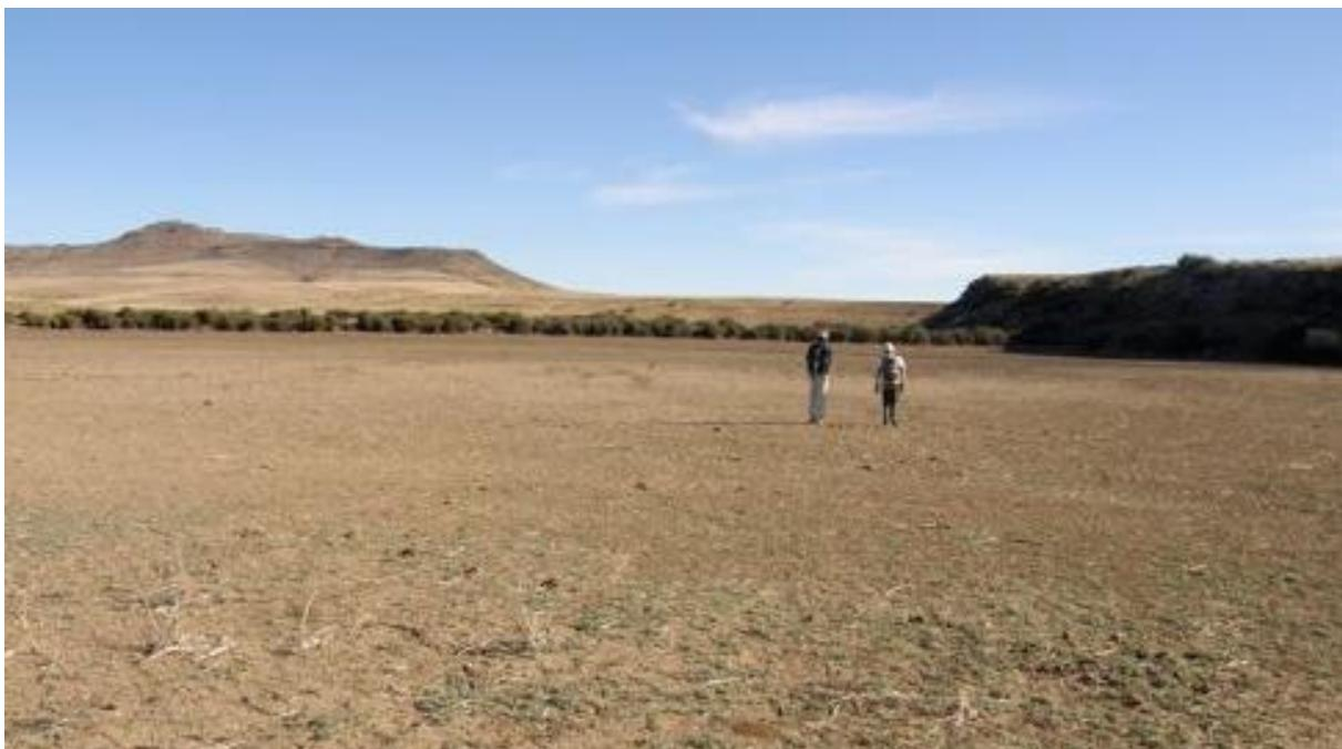
**Figure 4.2 Ganora Dam, a much smaller farm dam in the region, has been so impacted by siltation that it is empty at regular intervals (Source: Kate Rowntree).**
